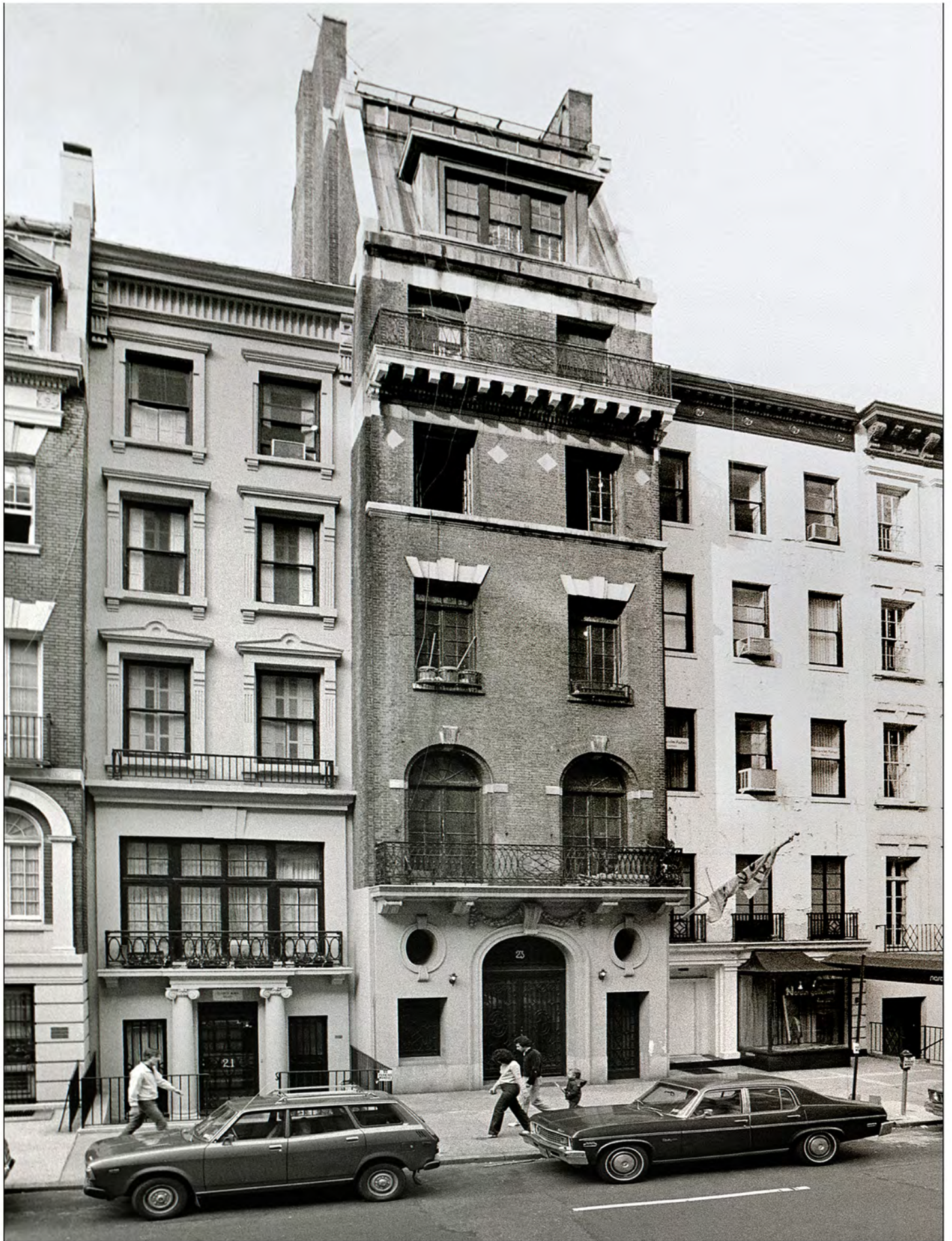
1977 | 23 EAST 73RD STREET STUDIO | PLATE N° 1 Insurance inventory photos documenting the Incredible Slidemakers studio.
